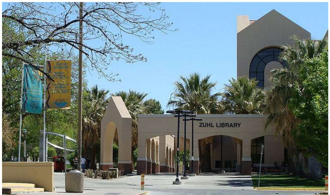
Zuhl Library at New Mexico State University (NMSU) in Las Cruces. © Wikimedia Commons
